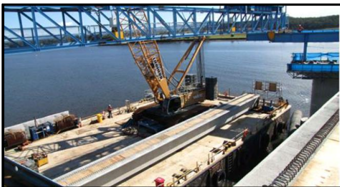
Side lifting truss
