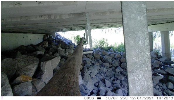
Plate 4.3 Northern bank at SBT2 with rock scour protection that crossing fauna need to navigate.
