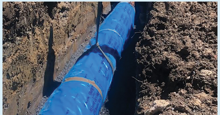
Water main relocation work has started at Stadium Drive
