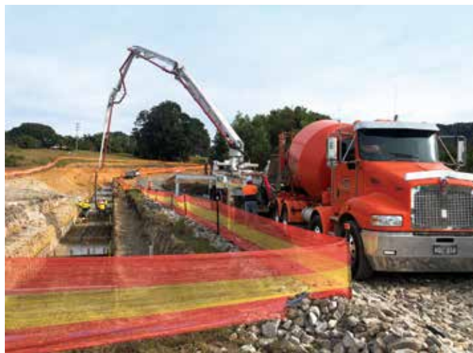
Preparing for the water main relocations on Coramba Road
