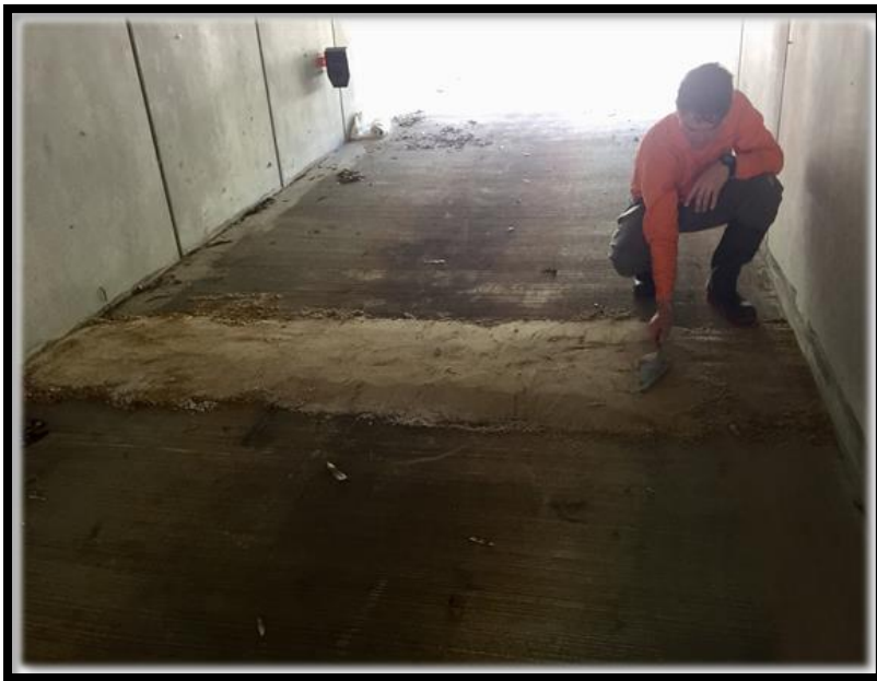
Plate 2: Sand pad installation at Tyson's underpass.
