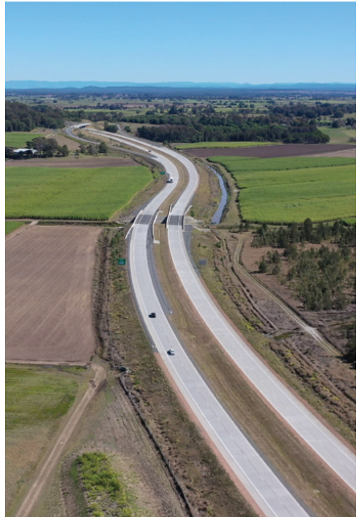
New motorway looking south toward Tyndale
