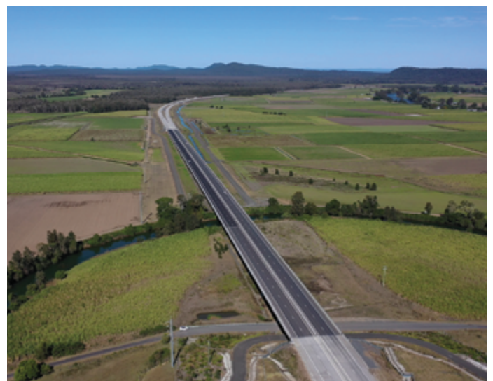
New bridge over Shark Creek
