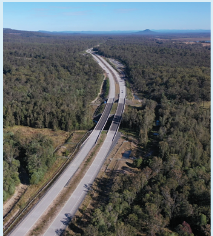
New motorway at Pillar Valley, looking south
