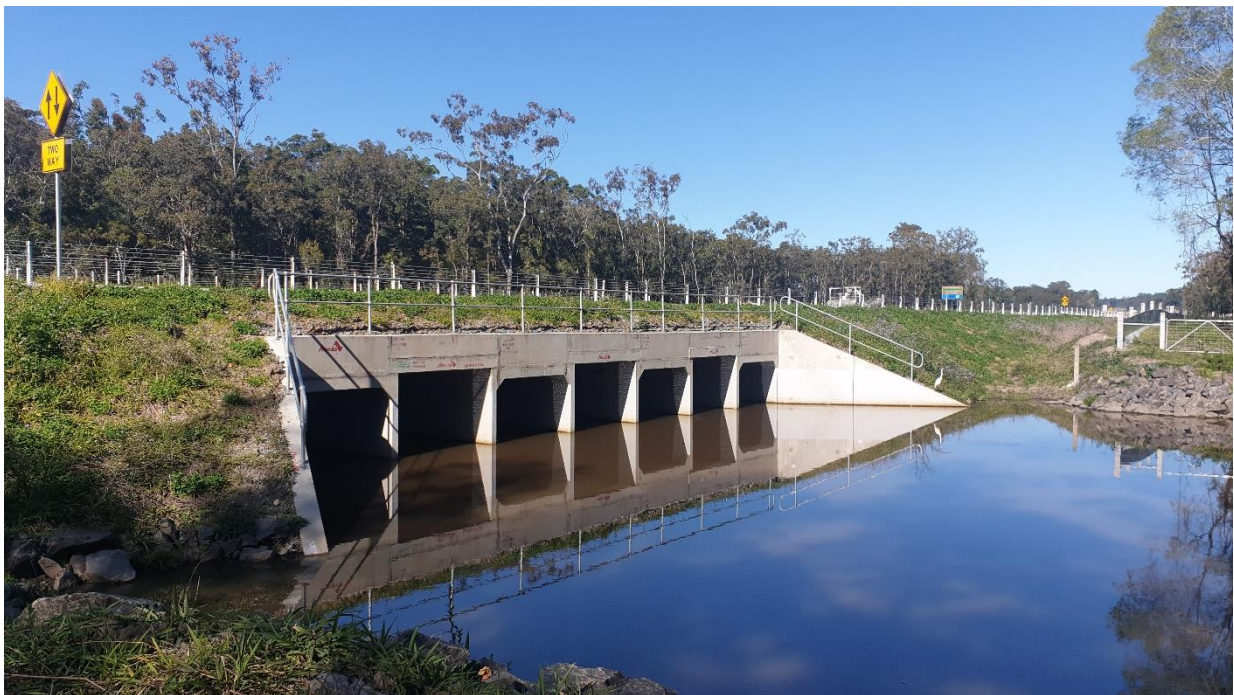
Plate 10: New Oakey Creek culvert, August 2020.
