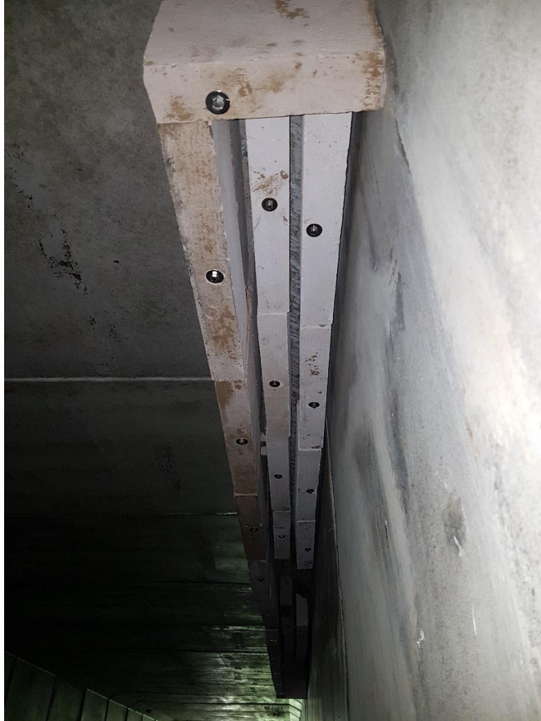
Plate 1: Prototype Hebel box designed to accommodate up to 2,000 Bent-winged Bats, installed in a box culvert at Glenugie CH 31400, March 2019.
