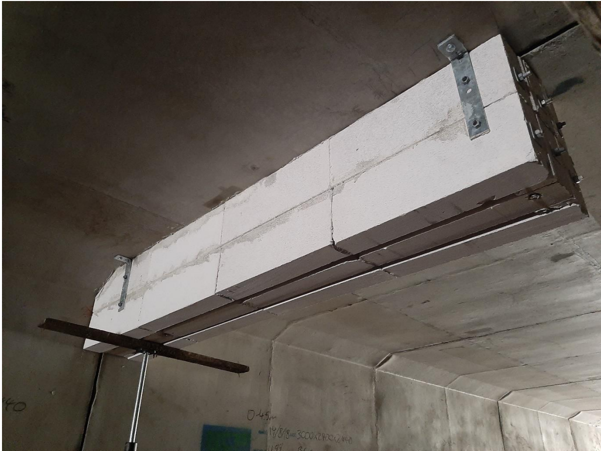
Plate 4: Large style double chambered Bent-winged Bat box constructed from Hebel blocks with capacity to accommodate hundreds of Bent-winged Bats installed in a box culvert beneath the Pacific Highway at Greenhill (CH 76400) in June 2021.
