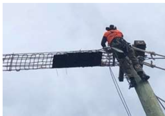
Plate 1: Rope bridges were suspended >10m above the road deck (upper) and supported by poles adjacent to the forest edge. A camera was strapped to the bulkhead at each end of the bridge (lower left). Black core-flute was cable tied to the underside of the rope ladder at each end during year 1 to reduce the incidence of false-triggering caused by traffic (lower right).
