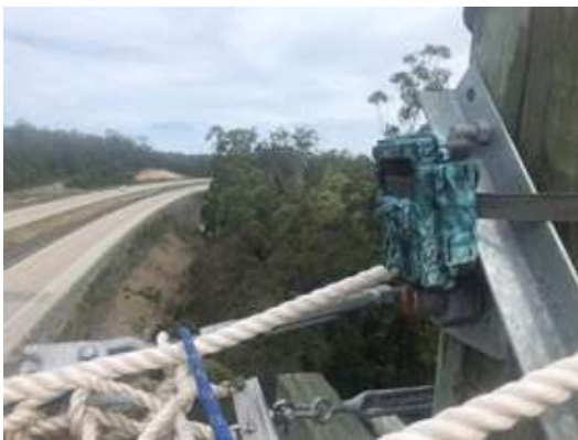
Plate 1: Rope bridges were suspended >10m above the road deck (upper) and supported by poles adjacent to the forest edge. A camera was strapped to the bulkhead at each end of the bridge (lower left). Black core-flute was cable tied to the underside of the rope ladder at each end during year 1 to reduce the incidence of false-triggering caused by traffic (lower right).
