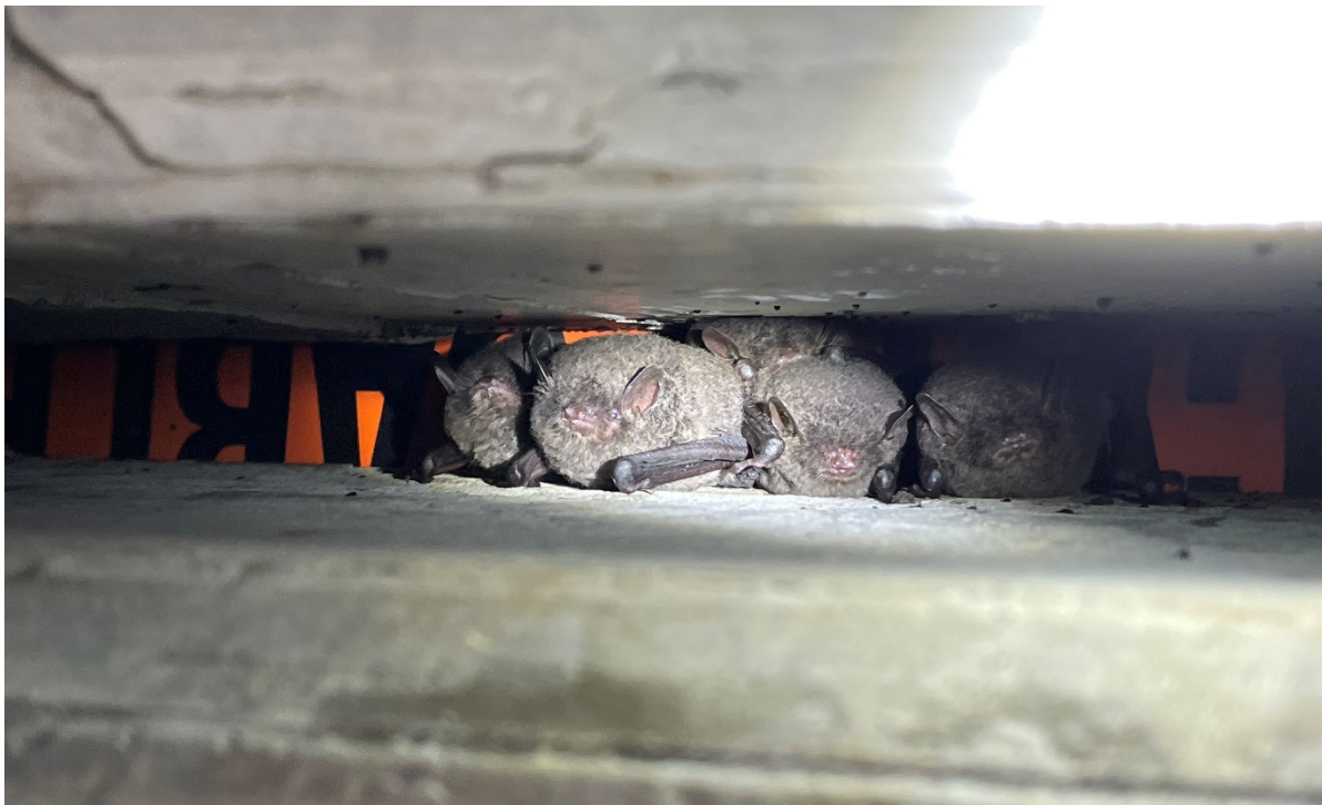
Plate 7: Myotis macropus roosting in culvert joints at site M36 in autumn/winter 2021.
