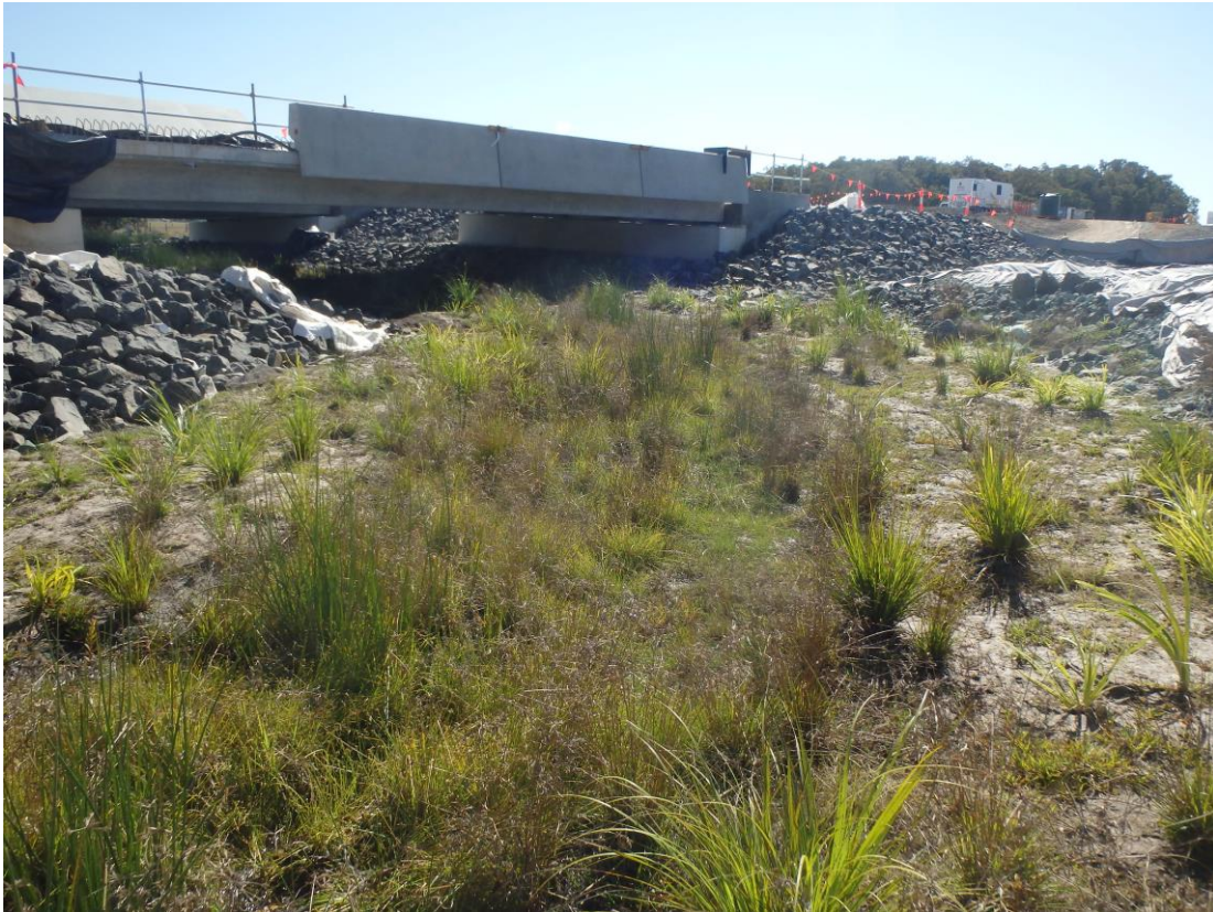
Plate 4.1 Site 13b in September 2018 after channel realignment and initial plant out.
