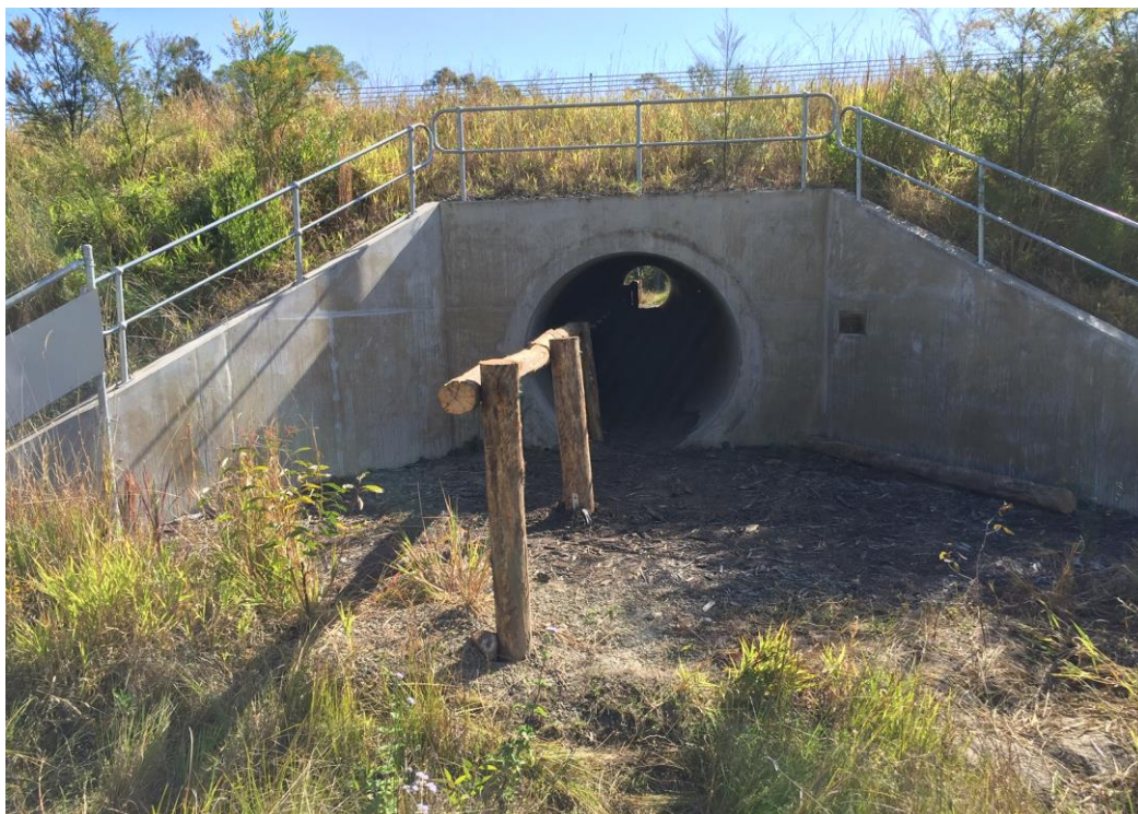
Figure 6 Fauna rail and refuge pole installed in fauna connectivity culvert.
