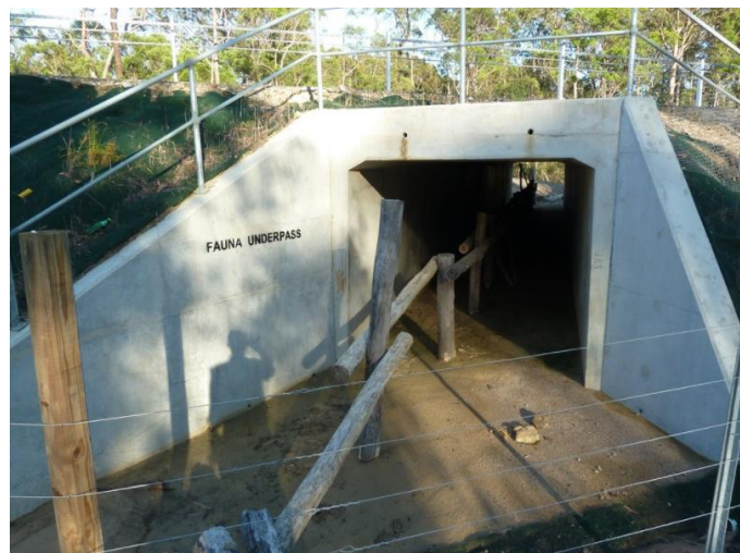
Figure 7 Wildlife protection, including Koala grids, signage, fauna furniture and culverts
