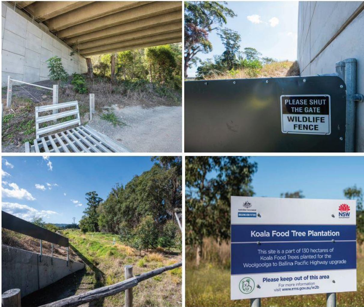
Figure 7 Wildlife protection, including Koala grids, signage, fauna furniture and culverts
