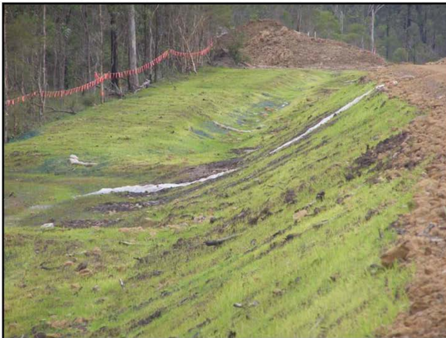
Plate 10: Successful establishment of cover crops on batters where mulch has been used with topsoil to assist temporary stabilisation.
