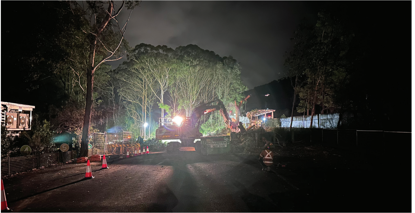
Night work for vegetation removal
