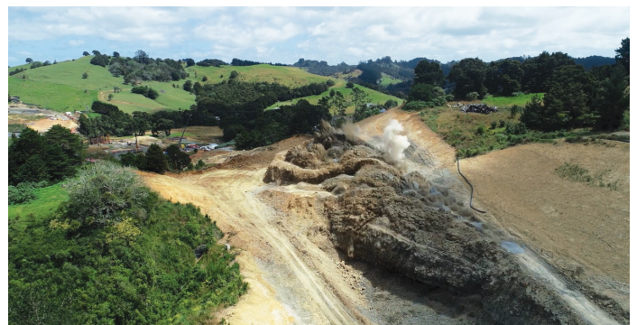
Controlled blasting at a cut site
