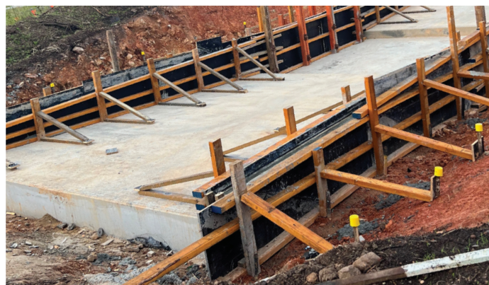
Construction has started on Panama disease wash-down facilities
