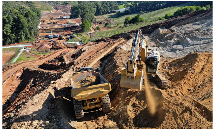
Excavator and Moxey in action near West Korora Road
