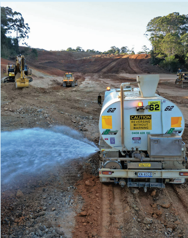
Water cart in action near North Boambee Road
