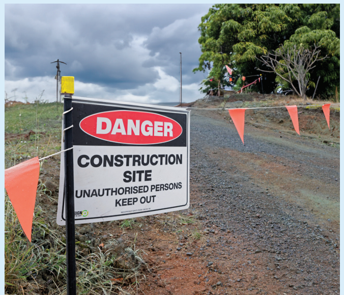
Delineation flagging and signage on site
