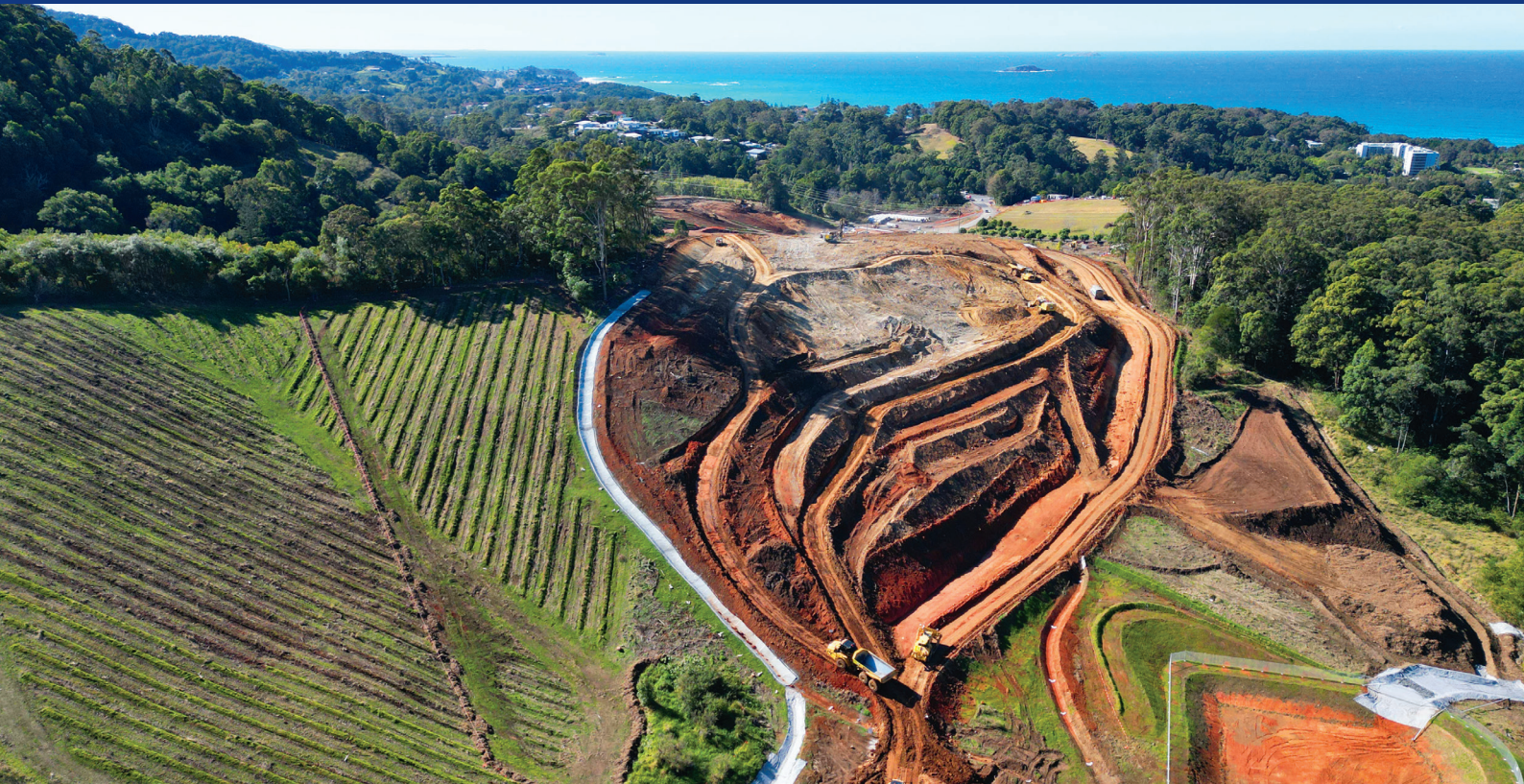
Cut site between Bruxner Park Road and West Korora Road
