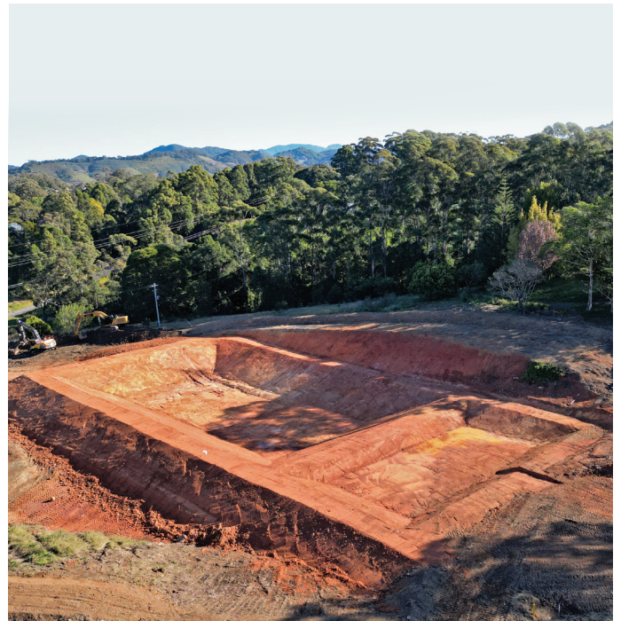
Sediment basin under construction near Mackays Road
