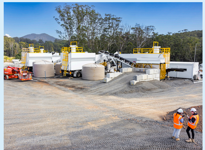
Batch plant on Englands Road
