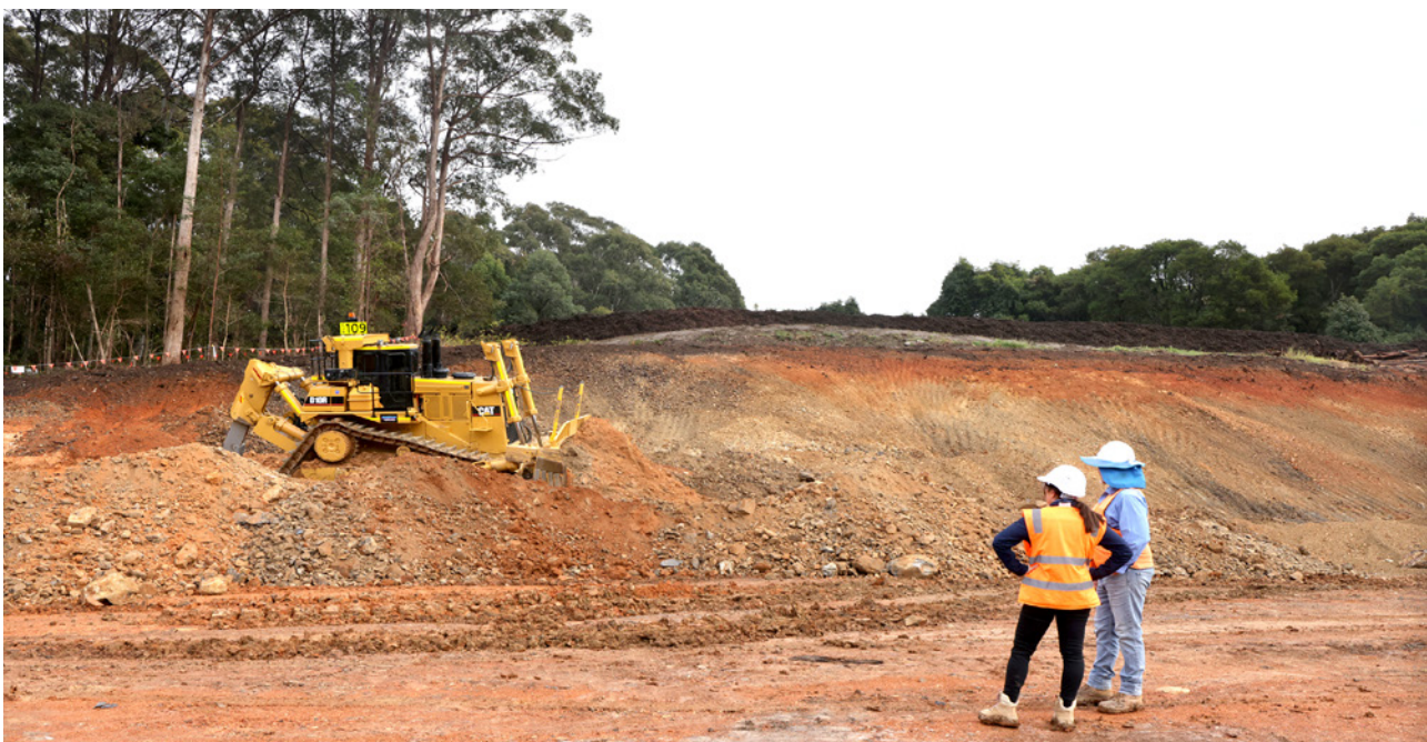
Project team supervising earthwork activities near North Boambee Road
