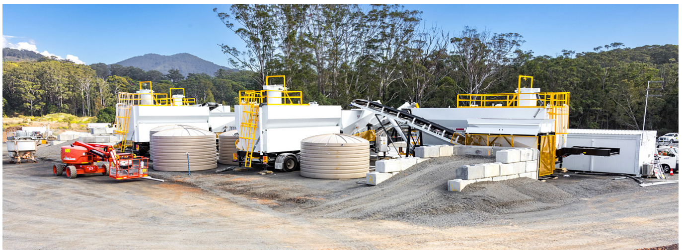
The Englands Road concrete batch plant arrangement
