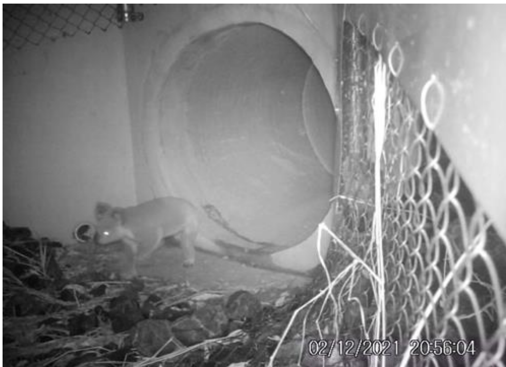
Plate 3: A koala was recorded making a southward crossing through a 1050mm wide by 15m long pipe culvert under Wardell Road on 2 December 2021.
