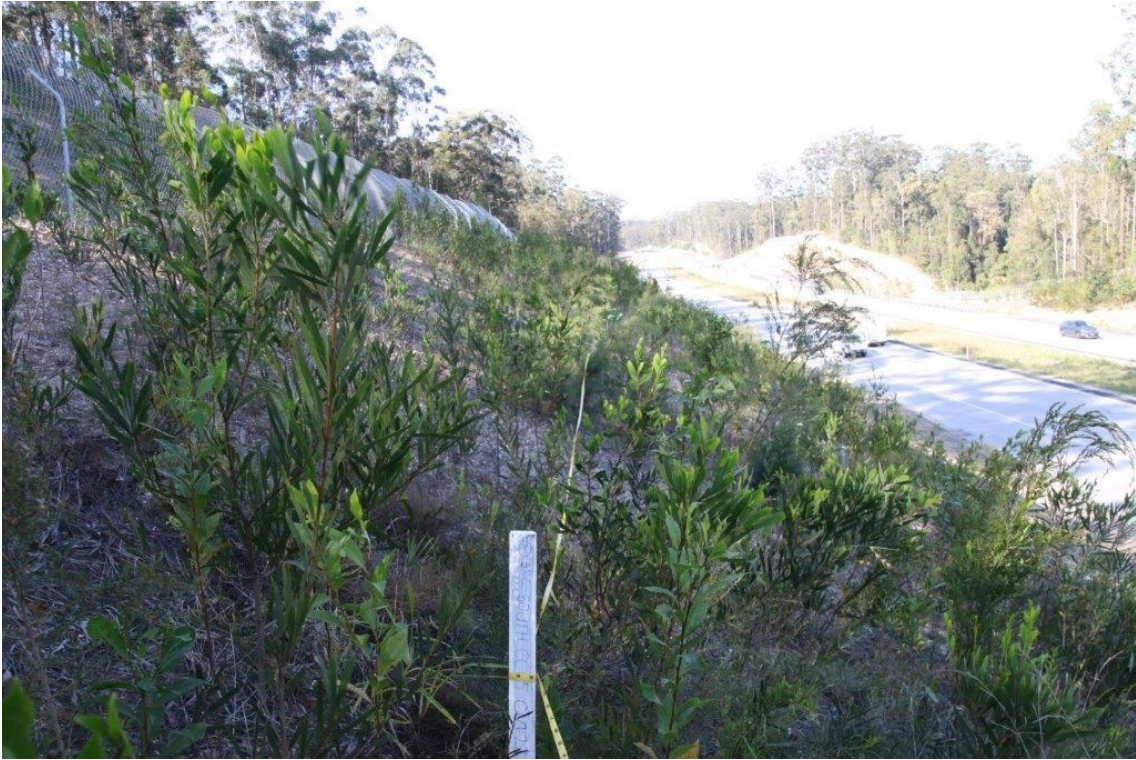
Spring 2018 - Site 7 southern end
