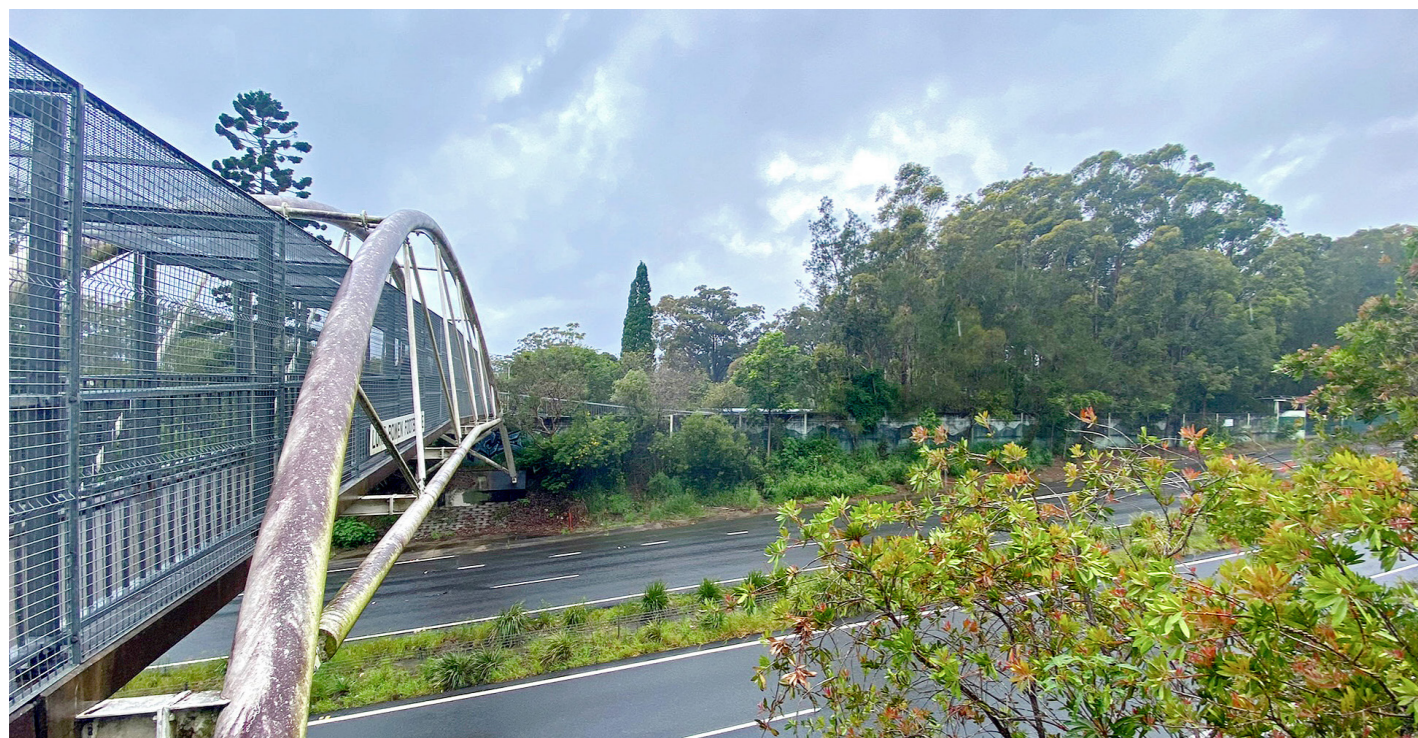
Figure 25: Luke Bowen Footbridge
