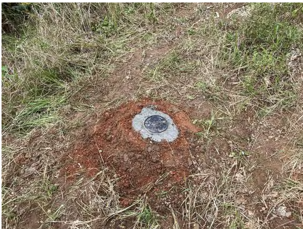
Photograph 4 , shows an example of a well repair for location BH2038, to the southeast of the Shephards lane tunnel.
