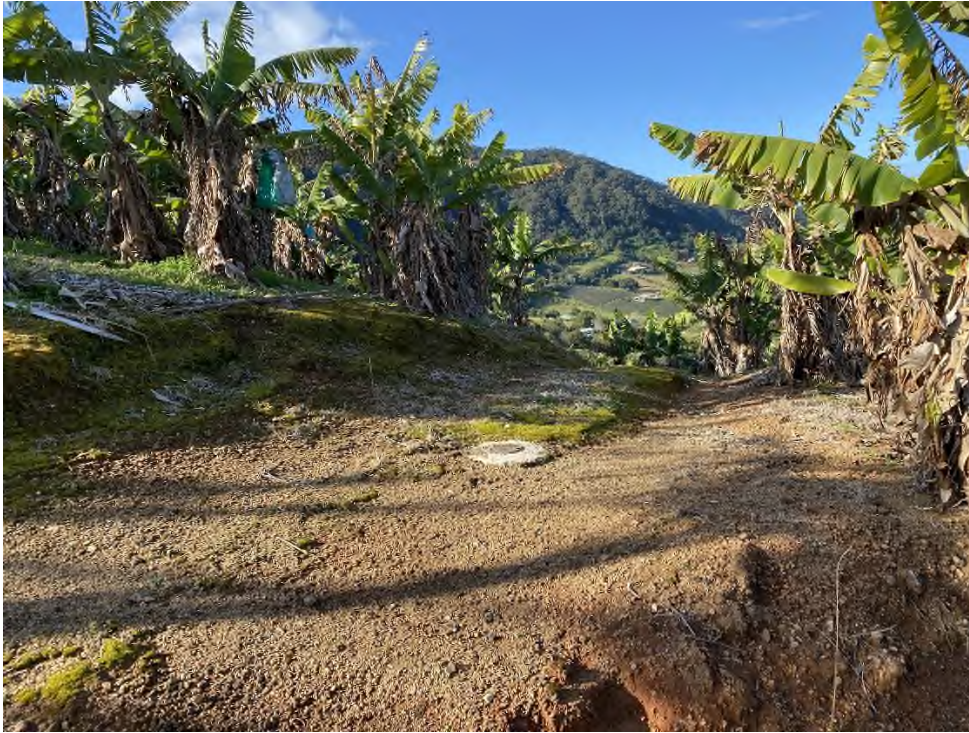
Photograph 1 , shows example of gatic cover installed at ground level in a banana plantation track. Location shown is BHH142 on ridgeline above Shephards Lane tunnel, view towards the northeast.
