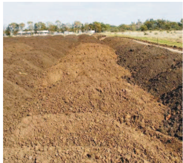
FIGURE 3.3: Topsoil being stockpiled at Moree for re-use later in revegetation and landscaping works (Photo: Lester Piggott).
