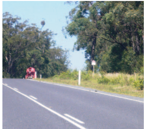
FIGURE 3.2: Natural regeneration occurred on Main Road 92 near Nowra, Southern Region after preparing ground with local soils and mulch (Photo: Gareth Collins).
