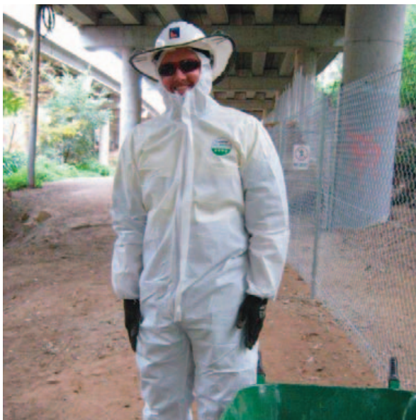
FIGURE 7.12: Disposable suits were worn on the M2 Upgrade Sydney Region when contractors were working in a positively identified Myrtle rust site adjacent to a critically endangered ecological community of Blue Gum High Forest. This level of hygiene is recommended when working in Myrtle rust sites that are adjacent to highly sensitive ecological areas (eg endangered populations and endangered ecological communities) (Photo: Donald Cheong).
