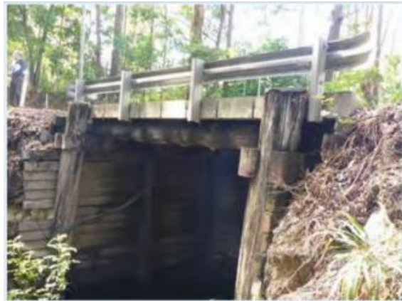
Photograph 6 Bridge concrete deck and under bridge
