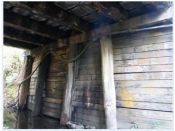
Photograph 5 Piles and sawn timber planks holding back the embankment
