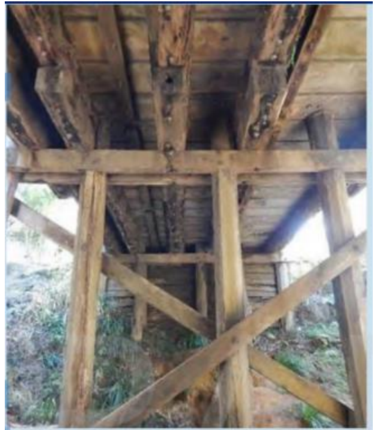
Photograph 3 Detail of the timber truss bridge
