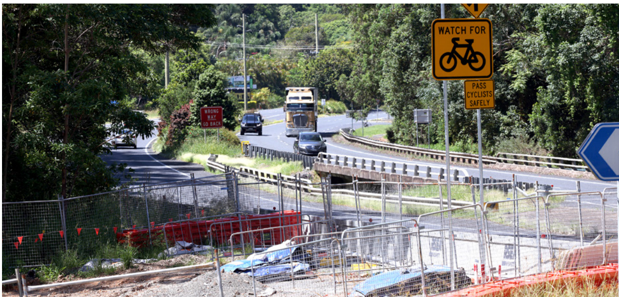
Utilities relocation work on the Coffs Harbour bypass
