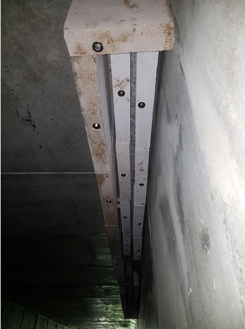
Plate 1: Prototype Hebel box designed to accommodate up to 2,000 Bent-winged Bats, installed in a box culvert at Glenugie CH 31400, March 2019.
