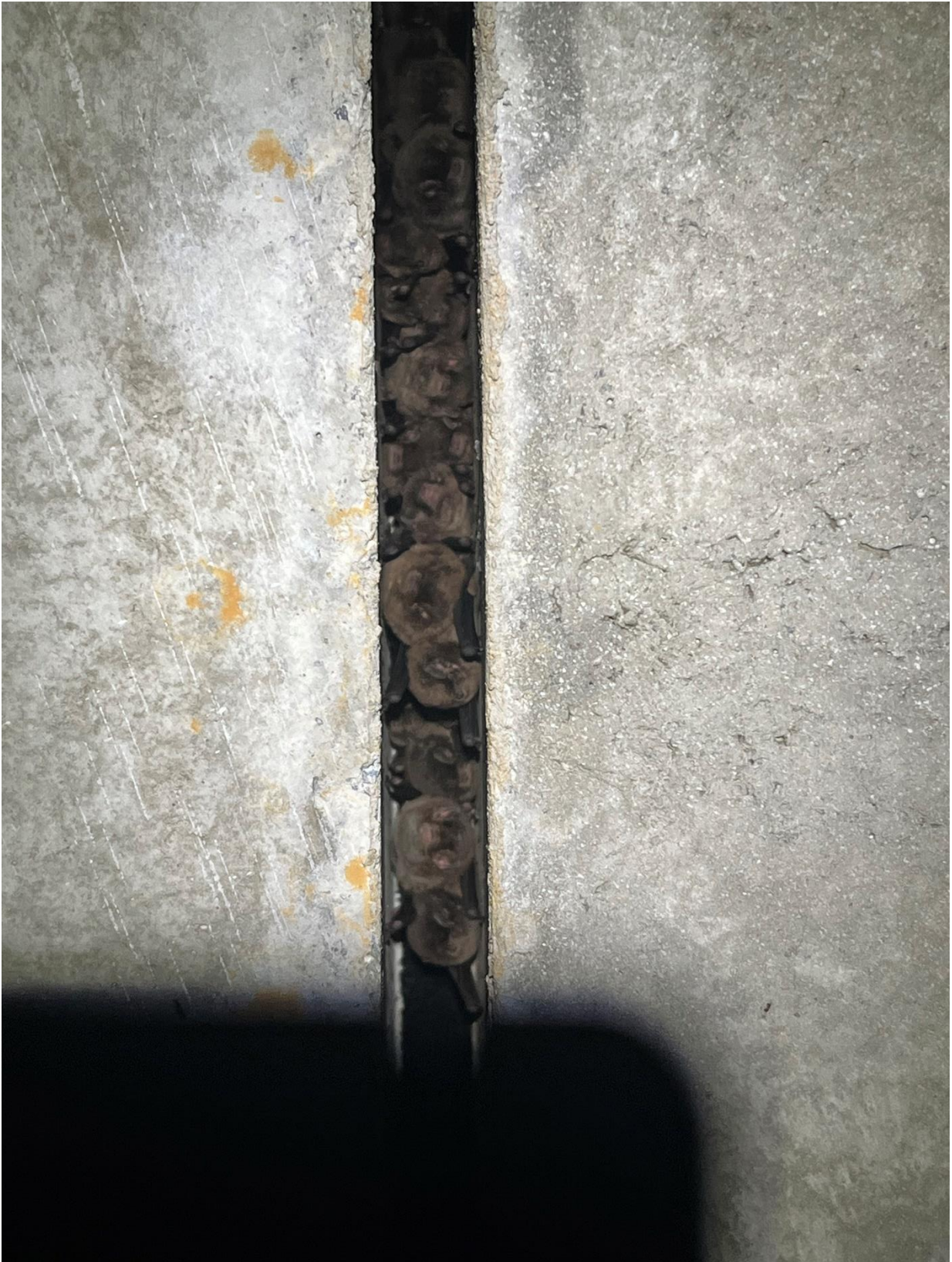
Plate 9: Little Bent-wing Bats recorded at Greenhill Box culvert (CH 76450), August 2022
