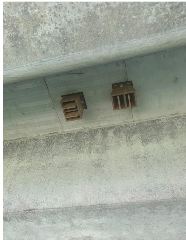
Plate 13: Two additional timbered four-chambered microbat boxes beneath Mororo Bridge (October 2023)
