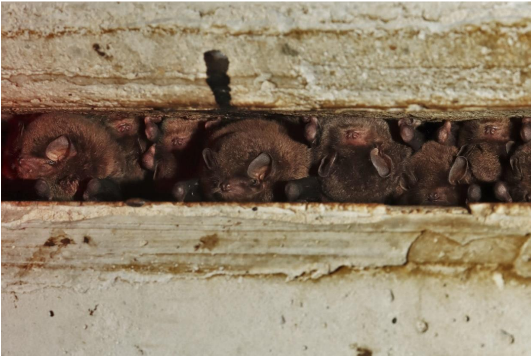
Plate 5: Little Bent-winged Bats at Glenugie Link Culvert (CH35075), August 2022
