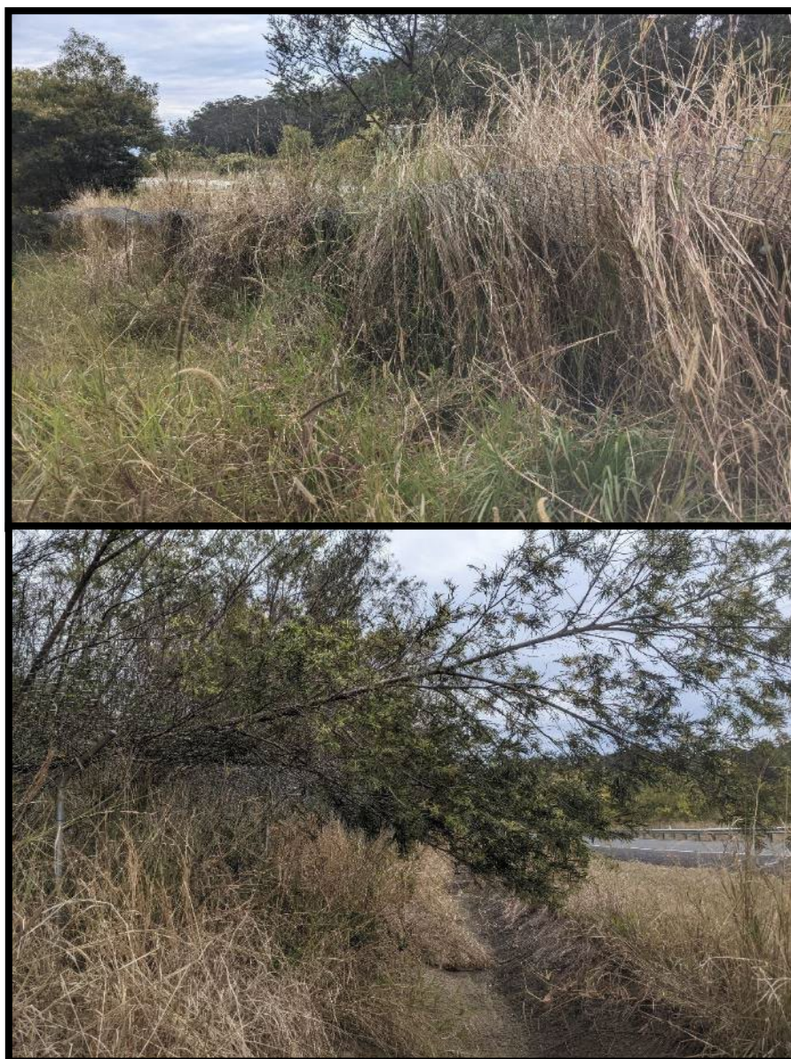
Plate 2: Thick grass protruding through and over the fauna fence north of Mattick Road (Top). Acacia spp. overhanging fauna fence adjacent to old coast road (Bottom).
