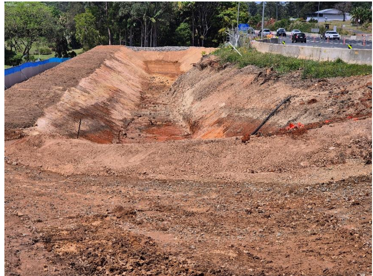
Image 8: Pacific Bay resort (Ch20900) – Sediment basin construction on east side of Pacific Hwy
