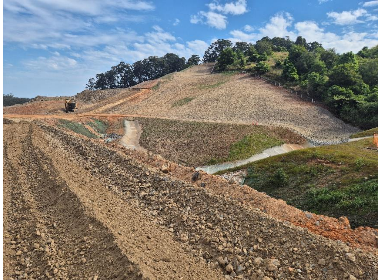
Image 4: Fill 4 (Just south of Roberts Road Tunnell South) showing rehabilitated (Ch13500)
