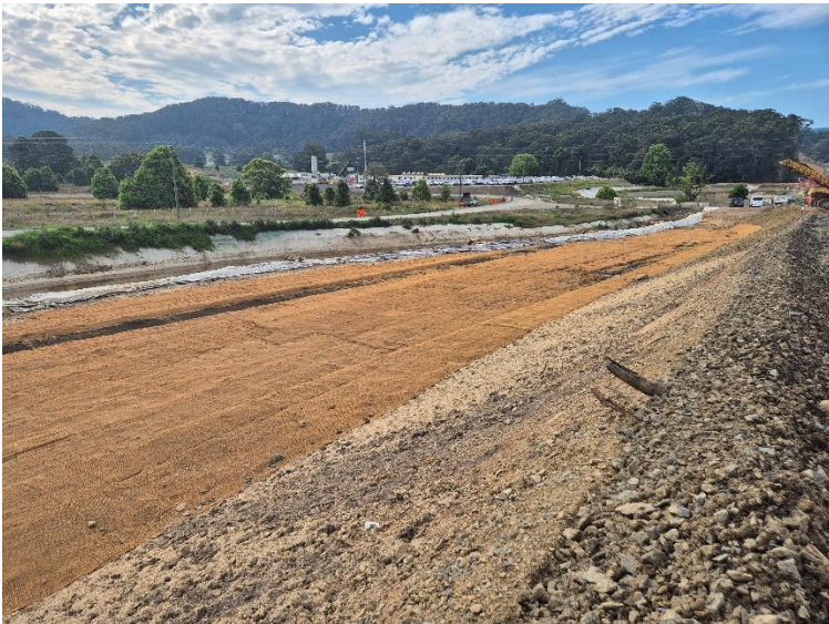
Image 3: Enlands Road at Fill 3B Redesigned and rehabilitated waterway (Ch12700)
