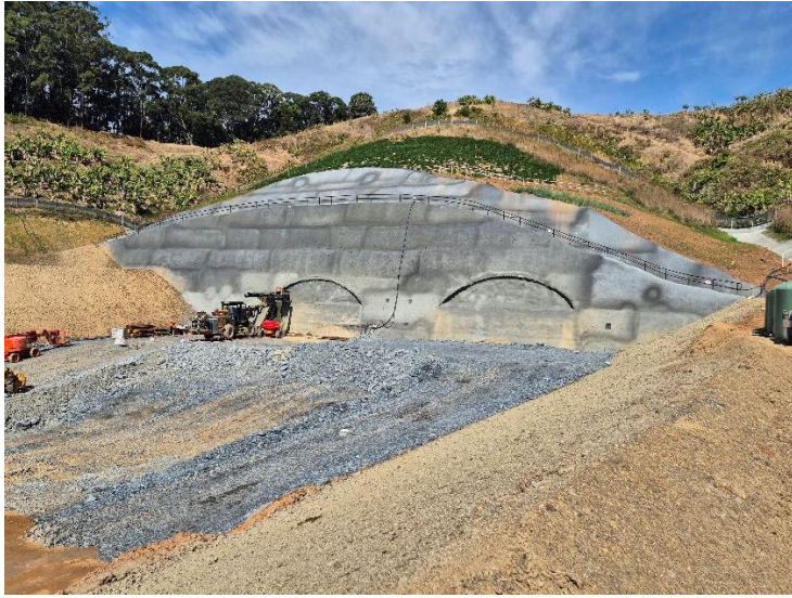
Image 5: Shephards Lane tunnel north portal (Ch17300) – Portal establishment and preparation for tunnelling
