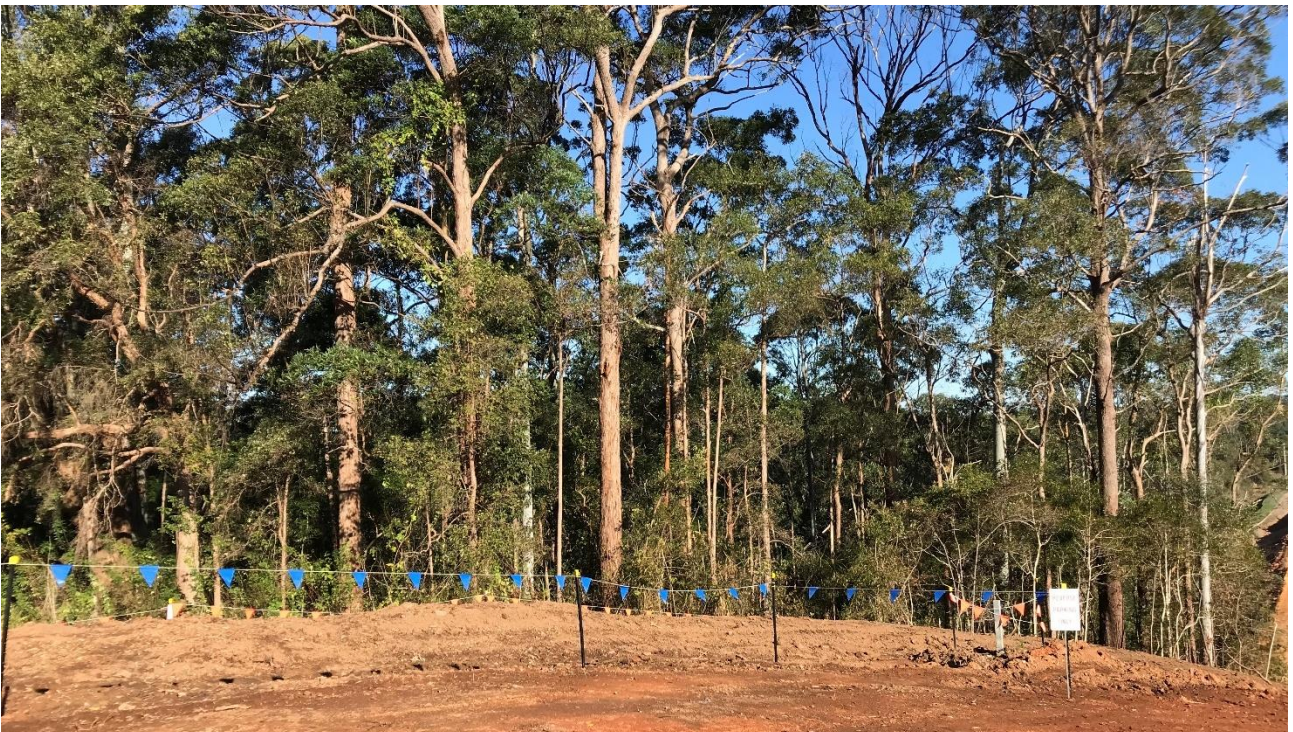
Photo 8 – Bunting indicating project boundary at Earthworks at Cut 4, Fill 3D worksite
