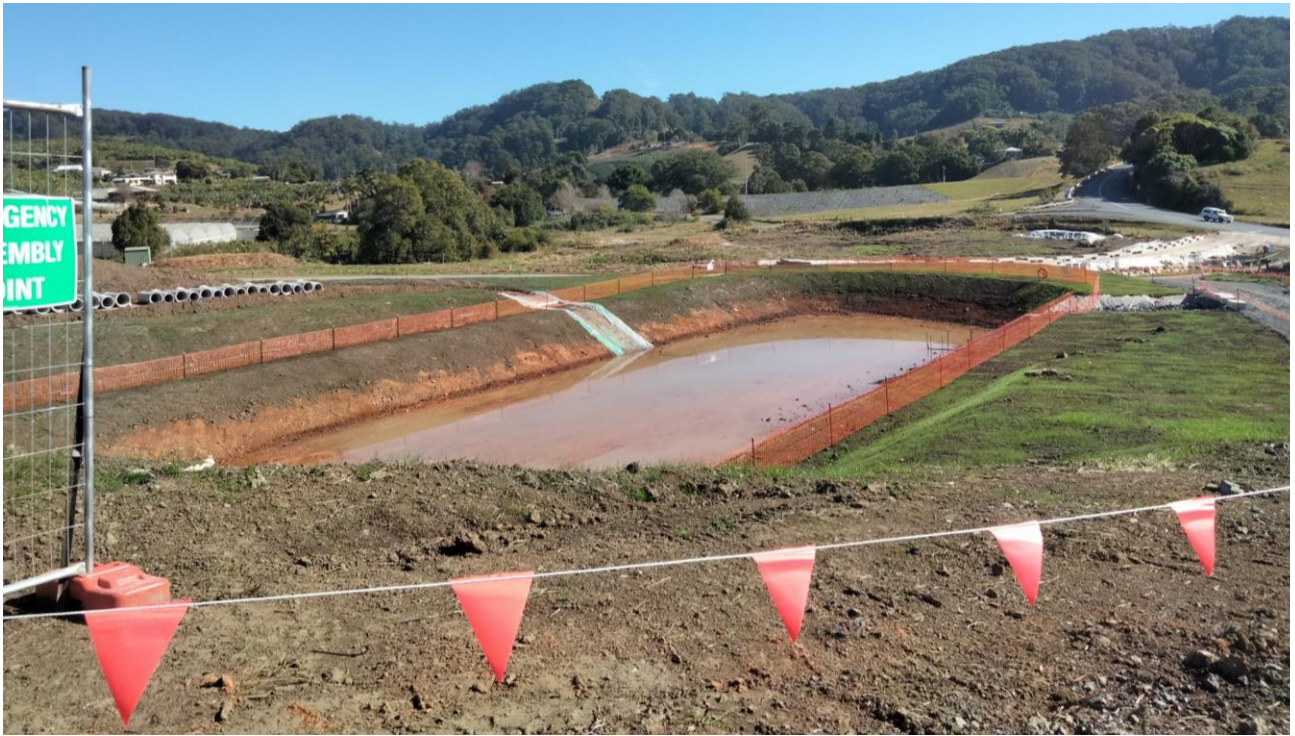
Photo 14 – Sediment basin at the South of Koramba Rd worksite
