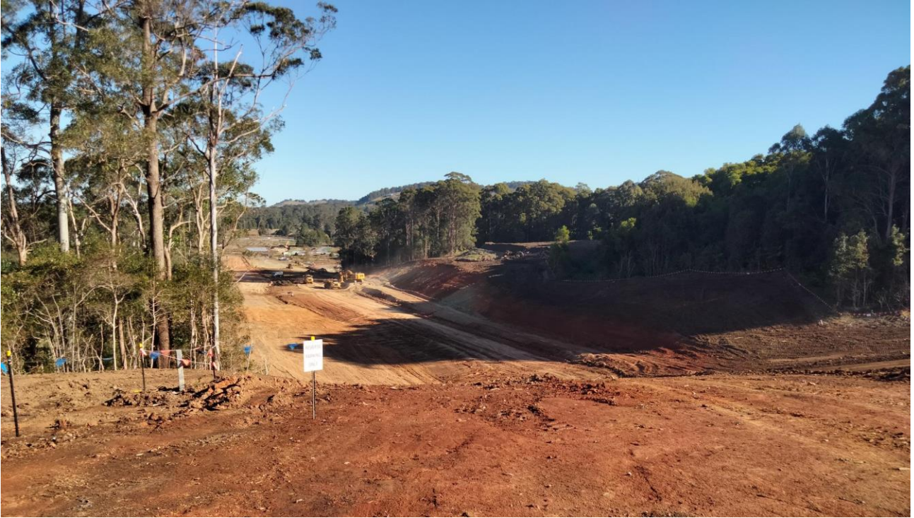
Photo 7 – Earthworks at Cut 4, Fill 3D worksite – note that dust is being generated and moving towards the project boundary in the photo
