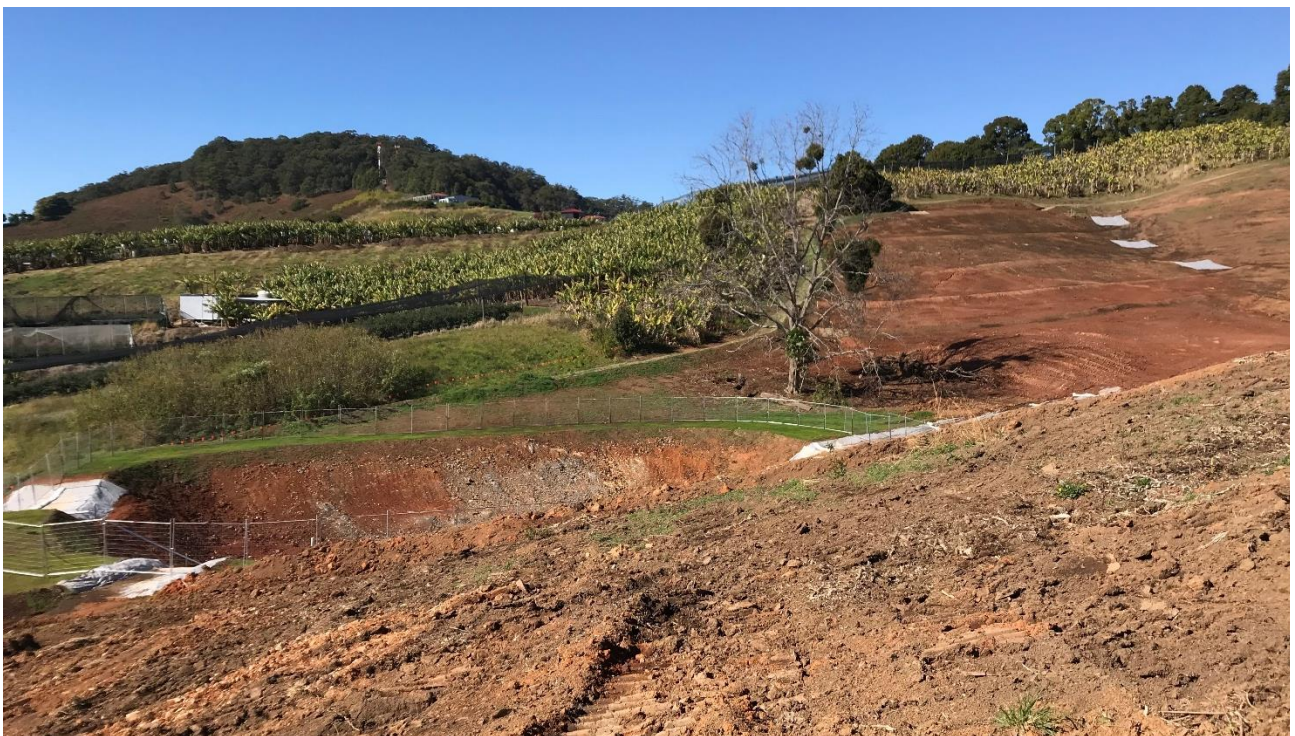
Photo 15 - Sediment basin and water diversions at the South of Koramba Rd worksite
