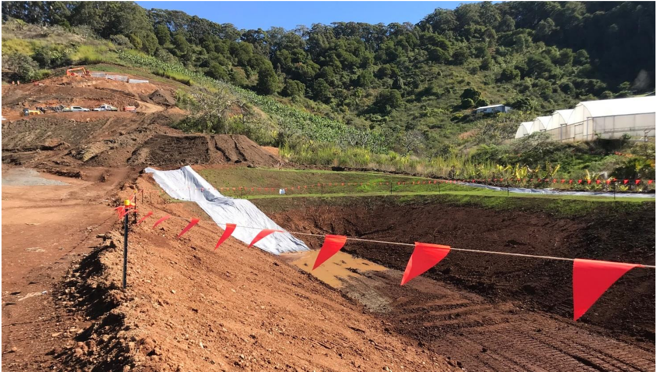
Photo 1 – Sediment basin at the West Korora Rd worksite
