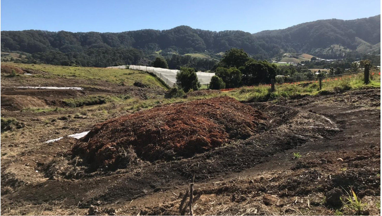
Photo 16 – Mulch stockpile surrounded with earth bund at the South of Koramba Rd worksite
