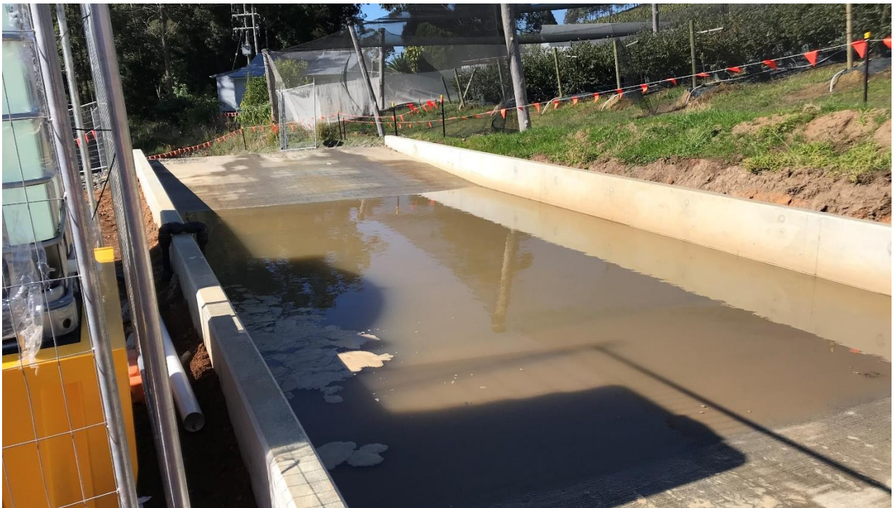
Photo 2 – Panama disease control wheel wash into West Korora Rd worksite
