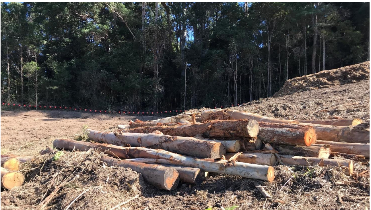
Photo 17 – Timber pins for reuse at the North of Koramba Rd worksite
