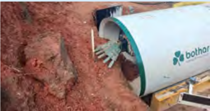
Mini tunnel boring machine clawing through the dirt
