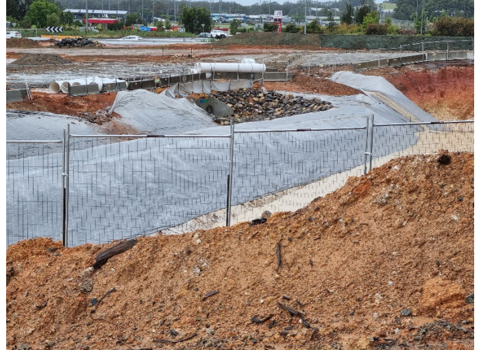
Image 2: Englands Rd Interchange (Ch10800) – Runoff into sediment basin during 27/10 rain event
