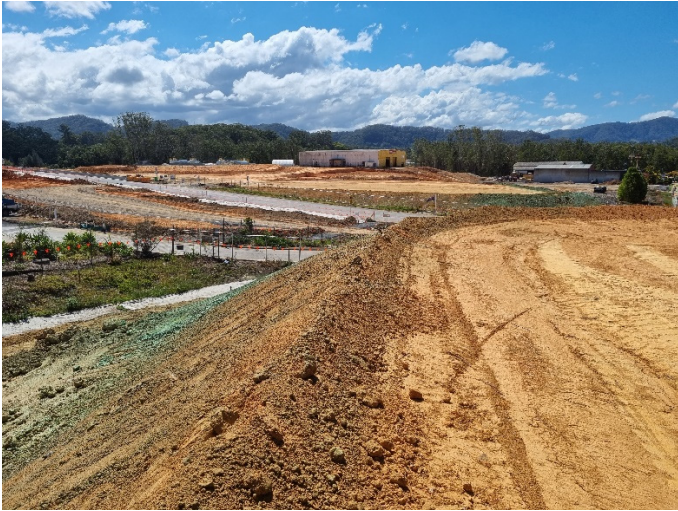
Image 1: Englands Rd Interchange (Ch10800) – Earthworks either side of Englands Rd
