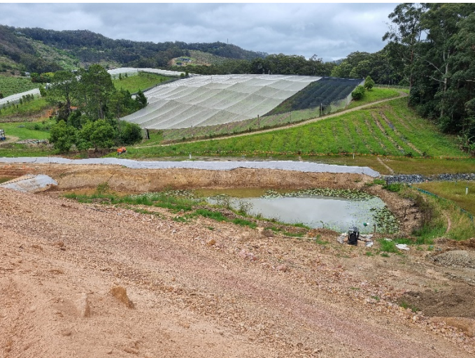
Image 7: Fill 18, Korora Hill (Ch21800) – Sediment basin construction and adjacent earthworks
