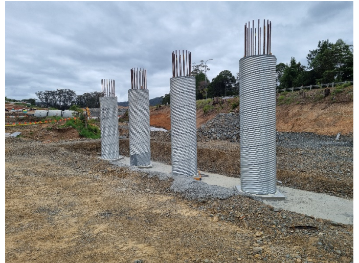
Image 6: Bruxner Park Rd / Pac Hwy intersection (Ch20900) – Bridge 19 piles
