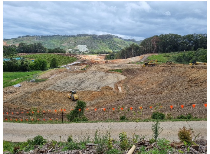
Image 2: Spagnolos Rd, Fill 8 (Ch15700) – Earthworks
