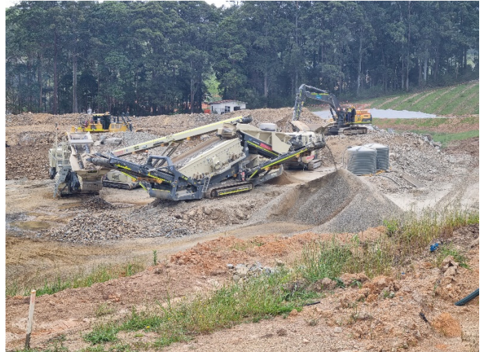
Image 4: West Korora Rd, north side (Ch19800) – Rock crushing operation
