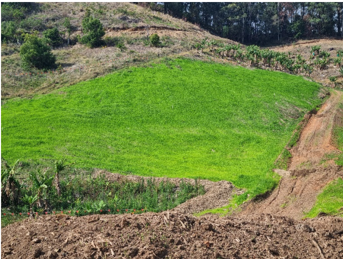
Image 3: Shephards Ln tunnel north portal (Ch17300) – Good establishment of cover crop following hydromulching
