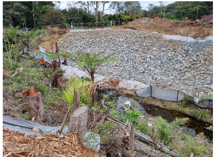
Image 8: Pine Brush Ck, Bridge 21 (Ch22300) – Installation of creek diversion
