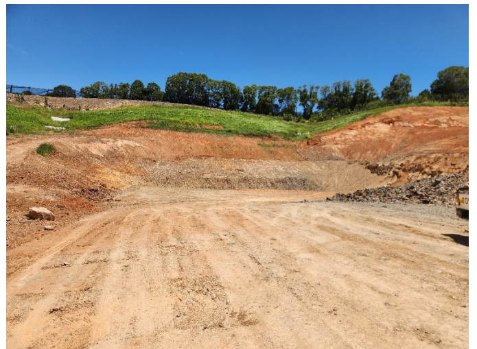
Image 4: Roberts Hill tunnel north portal (Ch13800) – Ongoing earthworks
