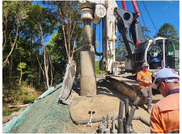
Image 2: North Boambee Rd, south side, Bridge 3 (Ch11700) – Bored piling
