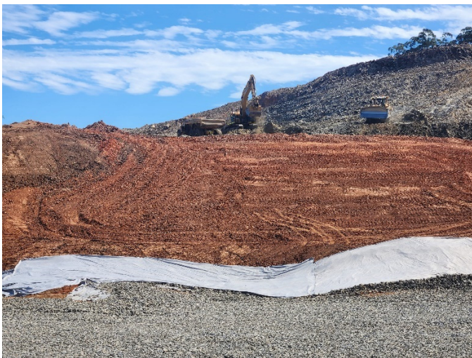
Image 3: Roberts Hill tunnel south portal, Cut 4 / Fill 4 (Ch13300) – Ongoing earthworks
