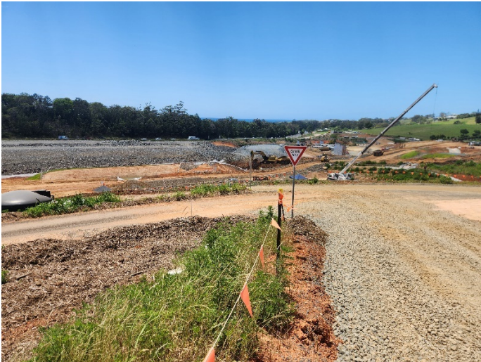
Image 7: Korora Hill Interchange, Fill 17 (Ch21000) – Earthworks and bored piling for bridges
