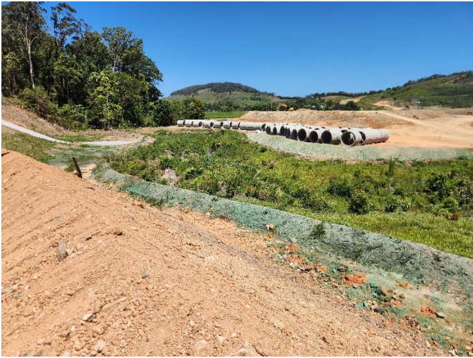
Image 5: Coramba Rd, north side, Fill 7 (Ch15200) – Preparation for cross-drainage pipe installation
