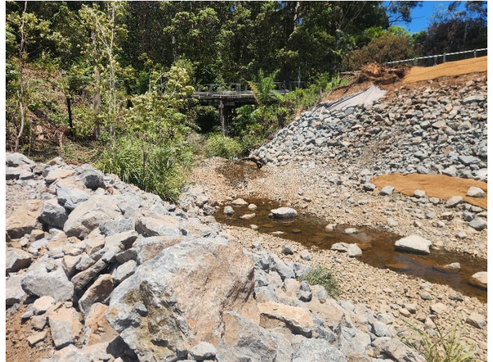
Image 8: Pine Brush Ck, Bridge 21 (Ch22400) – Installation of creek diversion
