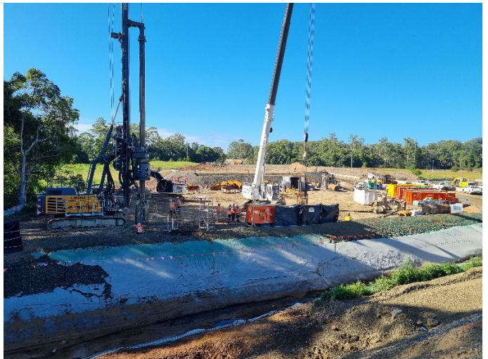
Image 4: North Boambee Rd, south side, Bridge 23 (Ch12000) – Bored piling
