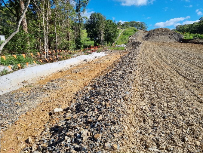
Image 1: Southern tie-in, Fill 0.5 (Ch9800) – Looking north along fill platform
