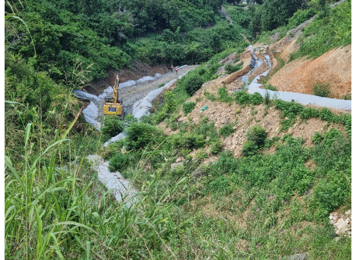
Image 6: Shephards Ln tunnel south portal (Ch16900) – Filling of gully
