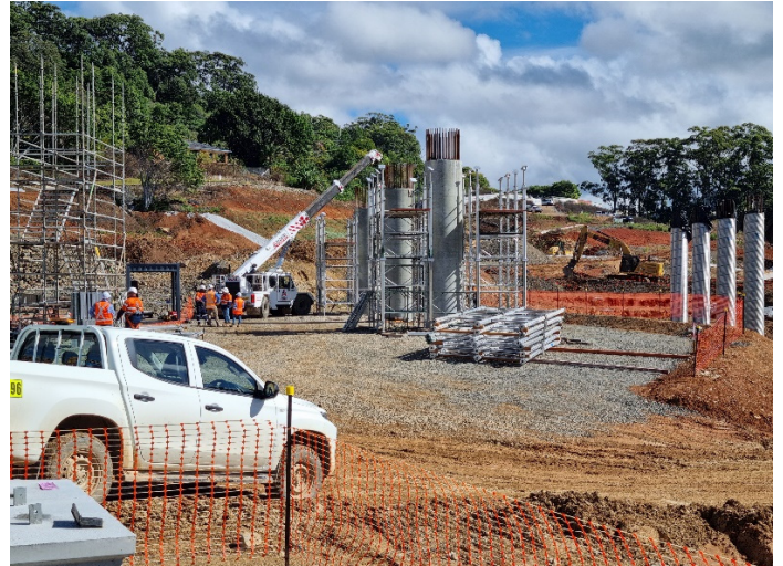
Image 8: Korora Hill Interchange, Bridge 19 (Ch20900) – Construction of bridge piers
