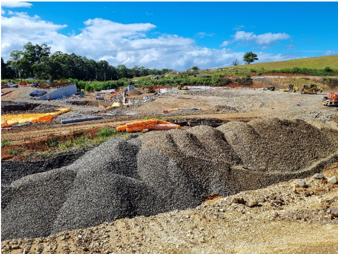
Image 7: Korora Hill Interchange, Fill 16 (Ch20800) – Looking south-east towards Bridge 18
