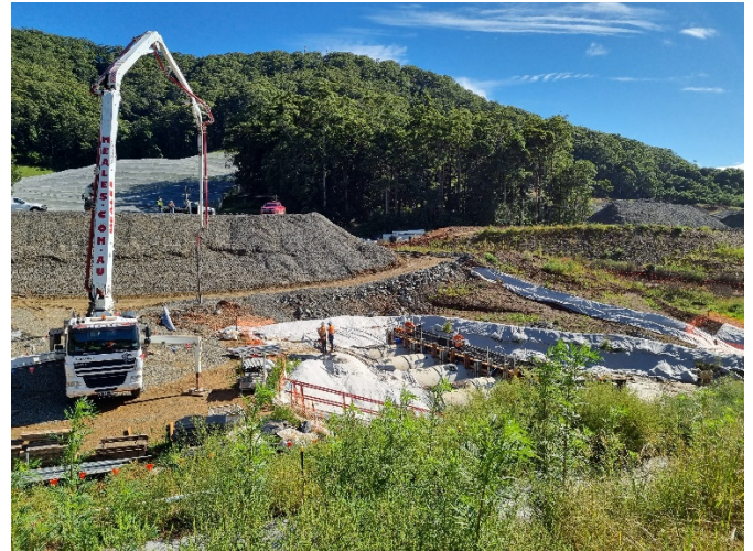
Image 6: West Korora Rd, Bridge 16 (Ch19600) – Pouring concrete headwalls on drainage culverts
