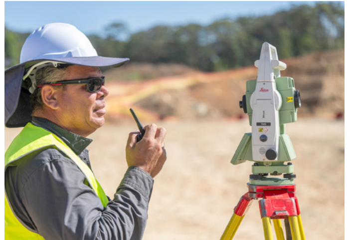
Surveyor assessing bridge columns at Korora Hill Interchange
