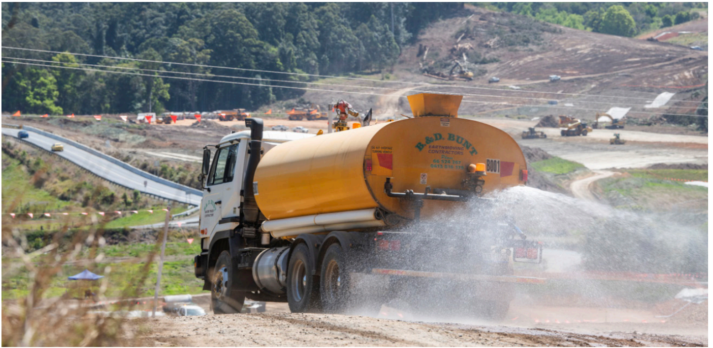
Water cart in action for dust suppression near Coramba Road
