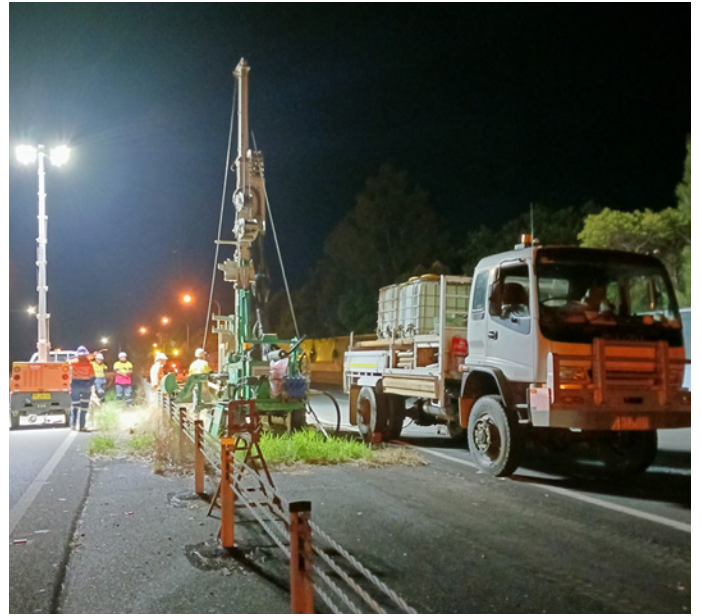
Geotechnical investigations being carried out in the median strip
