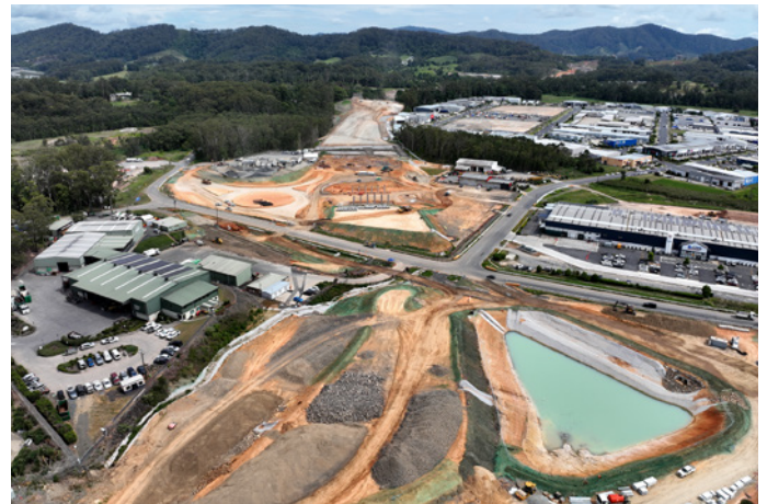
Earthwork operation at Englands Road Interchange
