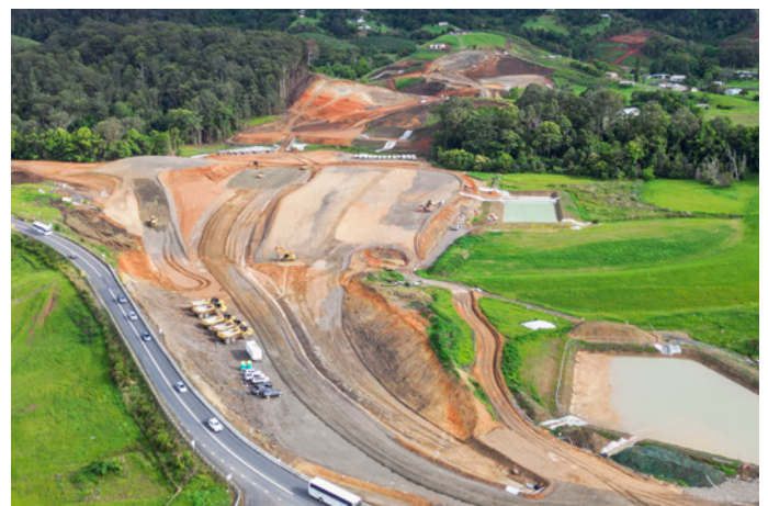
Earthwork operation at Coramba Road Interchange
