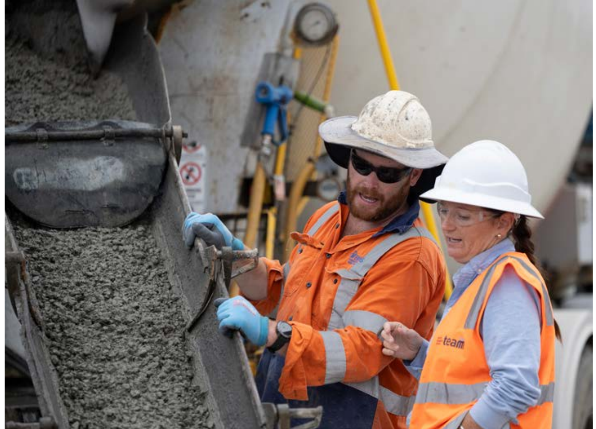
A tradesperson pours concrete while a project engineer examines the mix.
