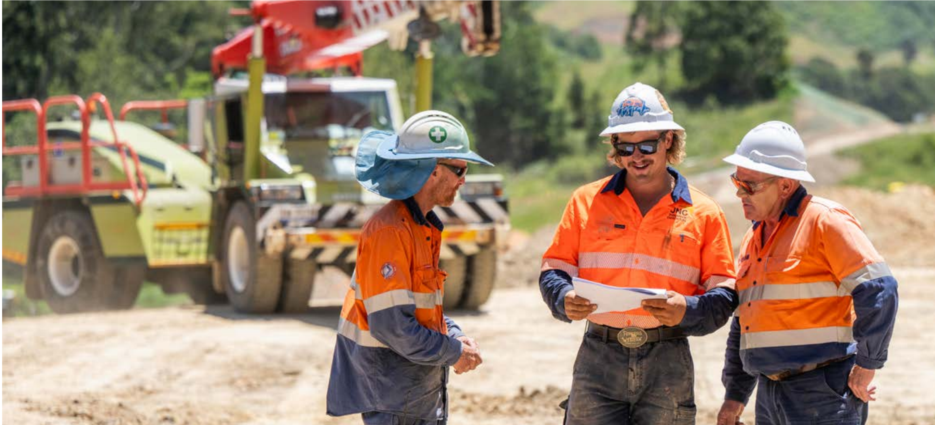
2 Skilled tradesman including from JNC Group (centre) at Gatelys Road Tunnel southern portal in January 2024. Gatelys Road Tunnel is the most developed tunnel along the bypass alignment (see pages 20-23).
