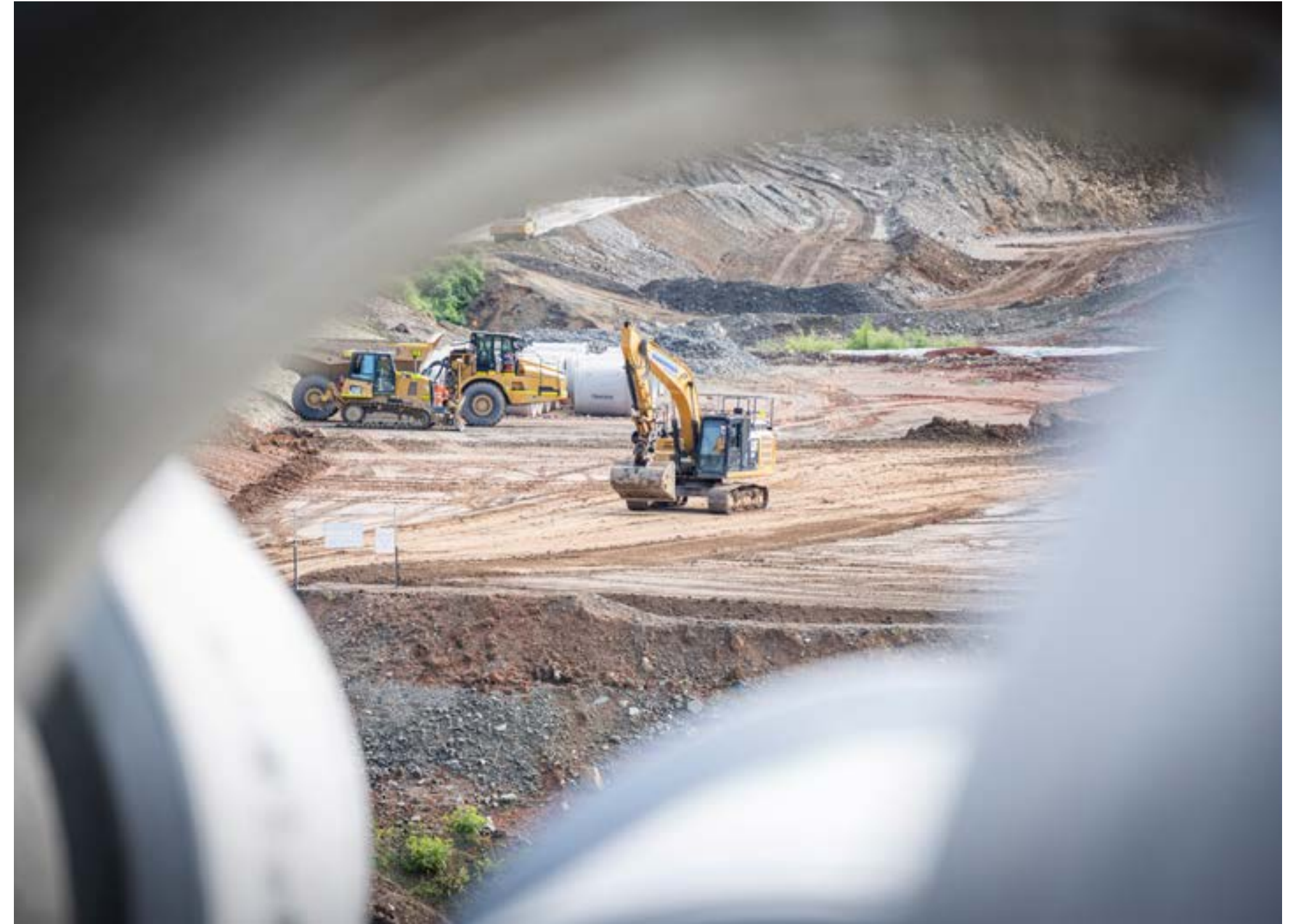
As at April 2024, 73 plant vehicles were mobilised to build the road.
