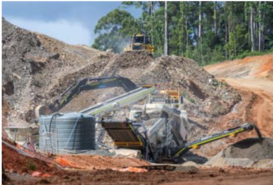
Above: north of Gatelys Road Tunnel is a deep earth cut – the largest required for the project. The earth is excavated in benches and its rock is crushed onsite, as pictured above.
