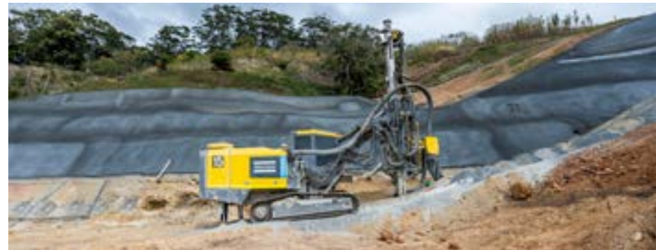
Above: the Coffs Harbour bypass' longest tunnel is Gatelys Road. Portal preparation work started in 2023 and progressed quickly, as pictures from (top) September 2023 and (top right) February 2024 shows. Right: a drill rig working at the tunnel portal.
