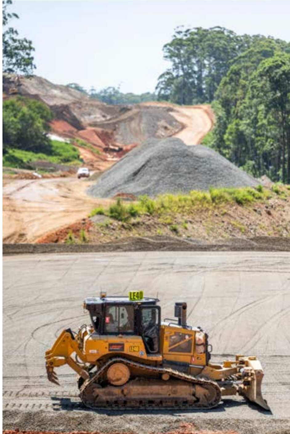
Above: north of Gatelys Road Tunnel is a deep earth cut – the largest required for the project. The earth is excavated in benches and its rock is crushed onsite, as pictured above.
