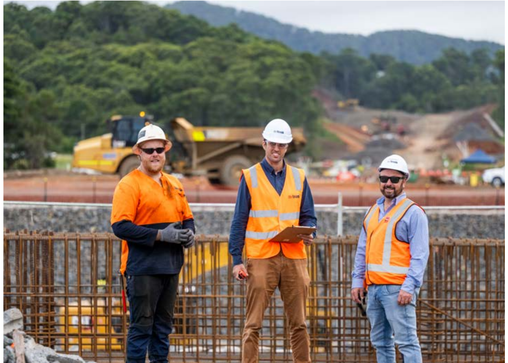
A skilled labourer and project managers from Transport for NSW and Ferrovial Gamuda Joint Venture discuss construction of the bridge.
