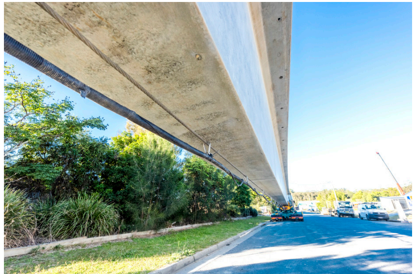
Underneath a Super T in place for an oversize, over-mass delivery.
