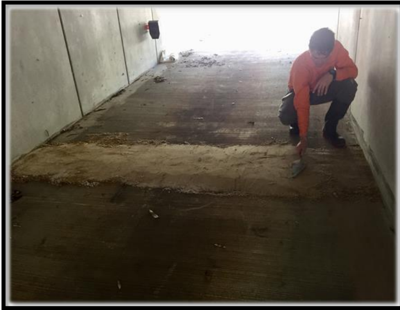
Plate 2: Sand pad installation at Tyson's underpass.
