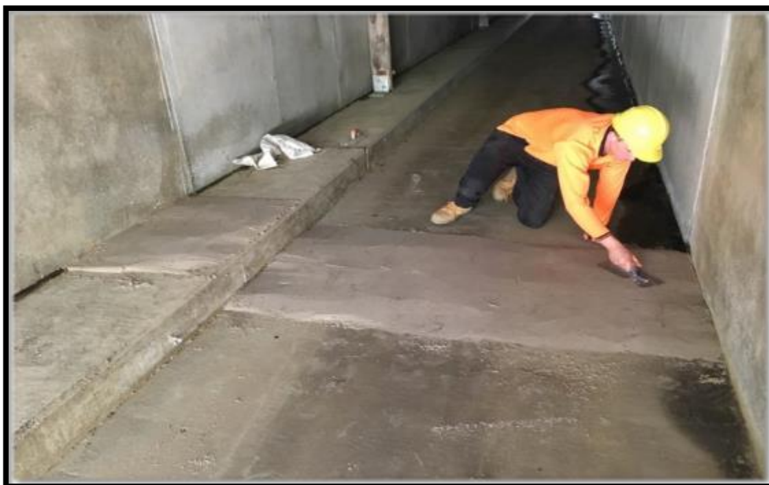
Plate 2. Sand pad being installed in a fauna underpass (Site 3) on the WC2NH upgrade.
